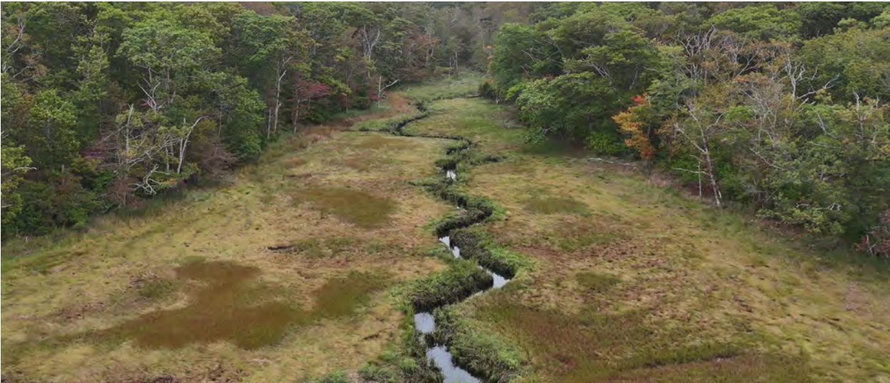
A culvert allows water to pass under Thatcher Road twice daily during high tides. This part of the marsh also receives water that drains down the slopes from higher points in Rockport.
